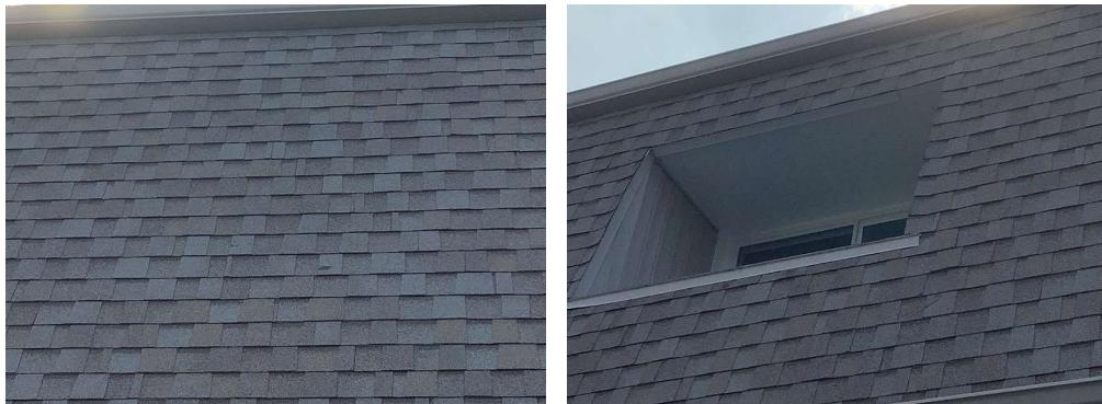
Mansard shingle roofing approximately sq ft. Data gathered from within the local market suggests a probable life cycle in the 20-25-year range for a professionally designed, installed, and maintained roof. The current cost estimate includes removal and disposal of the existing roofing, typical minor repairs to the underlying roof structures, flashing, etc., and installation of like roofing.
